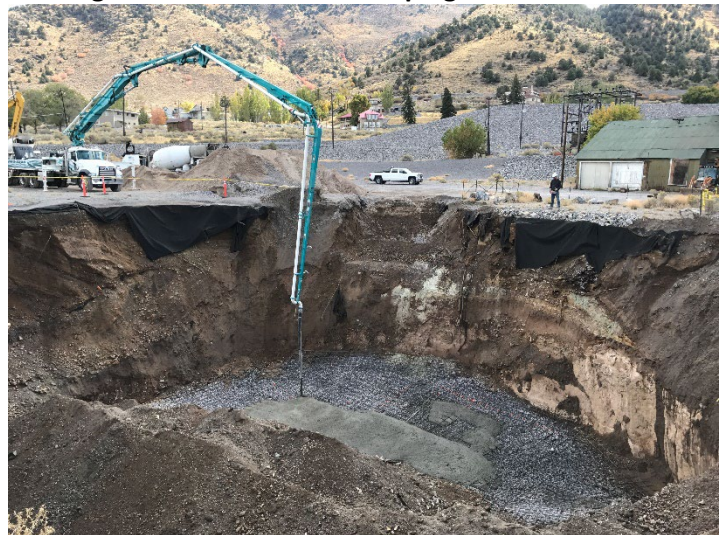
Backfilling the subsidence hole.
