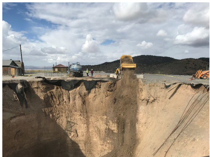
Backfilling the subsidence hole.
